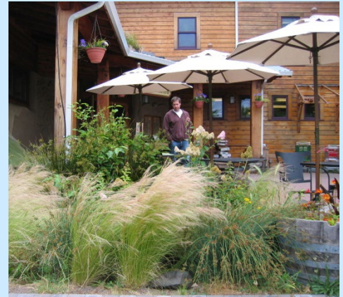
This rain garden collects roof water through a downspout.
