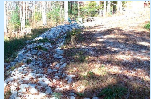
This diversion berm is constructed across a steep slope (max. 25% slope) to slow stormwater.
