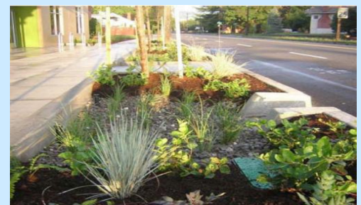
When this bioretention planter box is full of stormwater, the extra water "backs up" into the street to drain into a storm inlet. Source: ASLA HQs, Washington, DC
