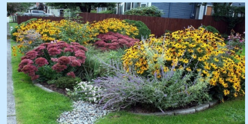
A stone channel is used in this residential rain garden to direct overflowing stormwater to the street. Source: Stewardship Partners/Flickr
