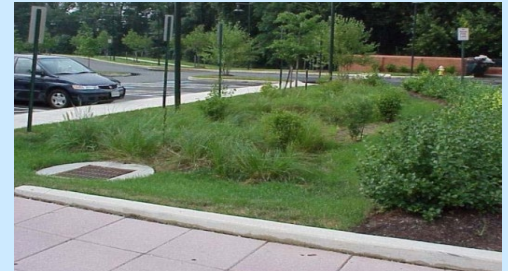
A storm inlet is used in this bioretention area to drain overflowing stormwater. Source: Pennsylvania Stormwater BMP Manual
