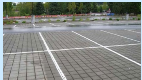
This large parking lot helps to infiltrate stormwater through a permeable pavement system.
