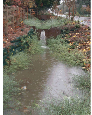
Cascading bioretention cells in Seattle help treat and infiltrate stormwater from roads.
